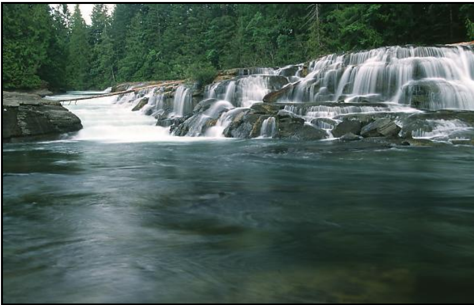
In-channel Rock Fishway – Stotan Falls, Puntledge River
