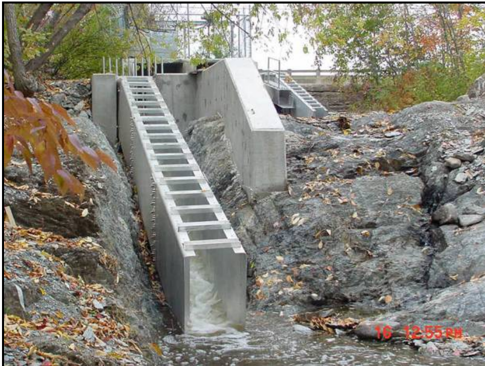
Alaska Steep-pass Fishway
